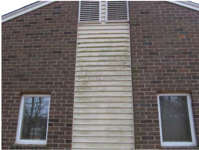
Dirt and organic growth typical on vinyl sided exterior wall surfaces
