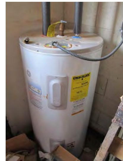
Electric, storage-type, domestic hot water tank for community building
