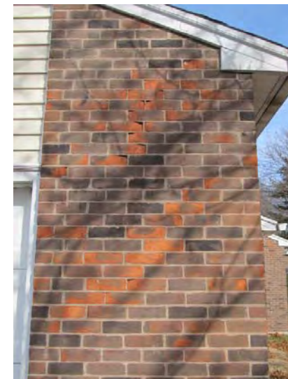
Areas of spalled brick noted at various locations throughout the development
