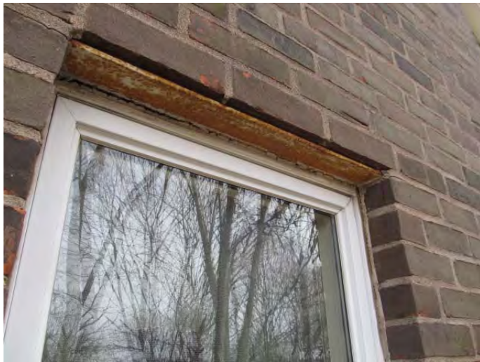
Steel lintels over windows and doors set in masonry openings are rusting and require surface preparation and painting in the near-term
