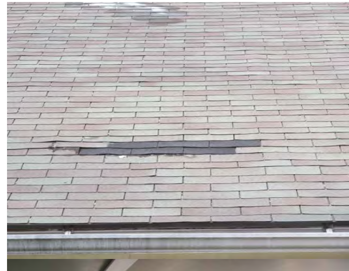
Roof shingles exhibit age and wear and have been patched at some locations
