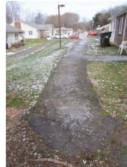
Original asphalt-paved sidewalks exhibit varying levels of wear and deterioration; some significant
