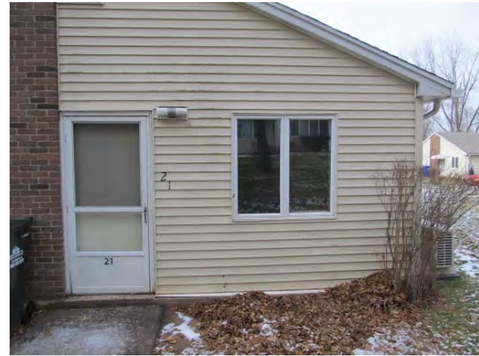
Typical unit entry door, storm door, and casement-style window – Most components exhibit age-related wear
