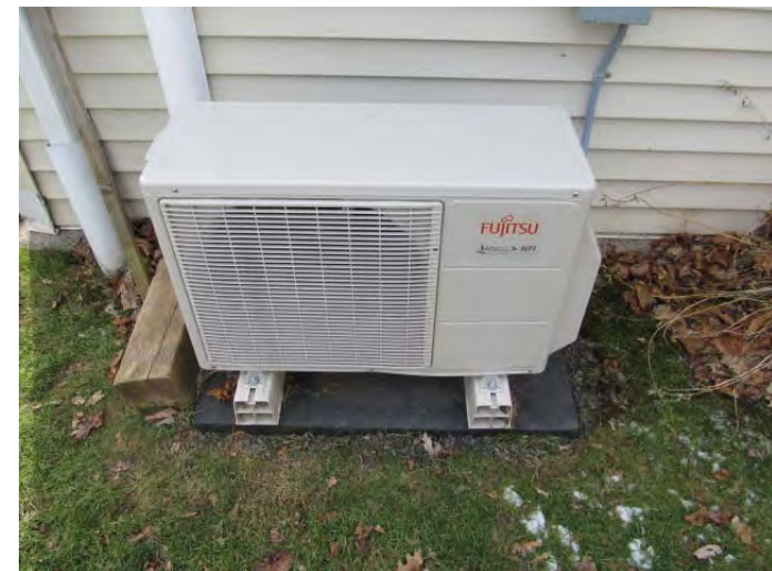
Typical exterior condenser for heat pumps that are found in all units
