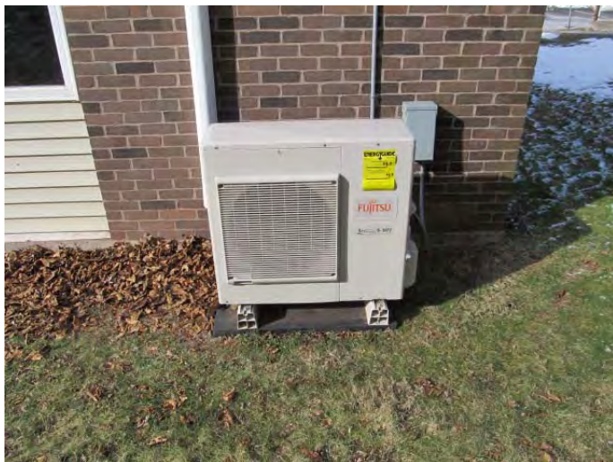
Exterior condenser for recently installed heat pump at community room
